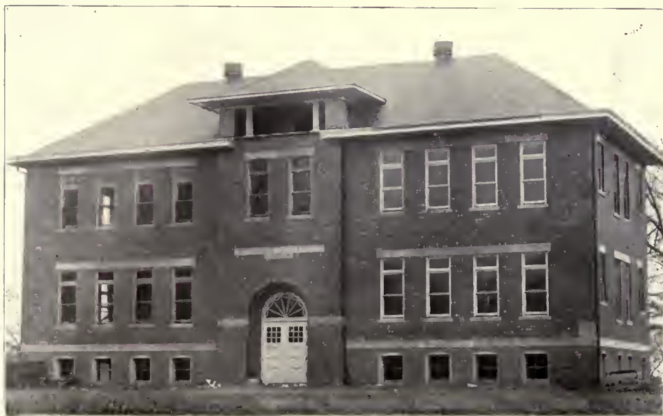
NEW HIGH SCHOOL BUILDING; PALMYRA
